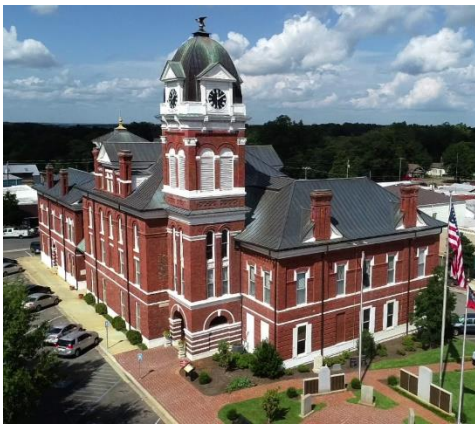
Aerial image of the Washington County courthouse Photo from http://washingtondev.com/
